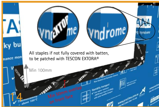
Applying TESCON EXTOSEAL® Sill Tape TESCON EXTOSEAL® Sill Tape should extend minimum 100 mm up the jambs. The corners of the TESCON EXTOSEAL® are stretched & adhered into place.
