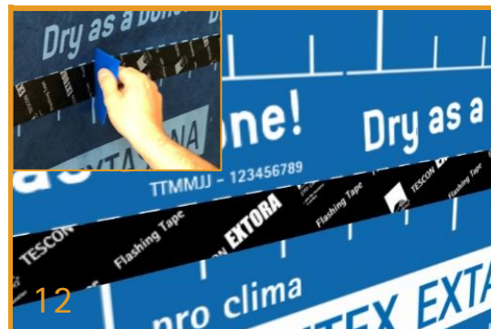
Connections Using TESCON EXTORA® Flashing Tape Apply at minimum TESCON EXTORA® 60 mm to the horizontal joints and apply pressure with the PRESSFIX tool.
