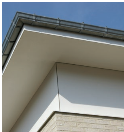
Roof finish in Cedral Board
