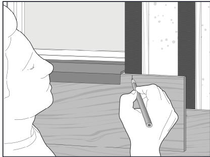
Mark the location of the plank.
