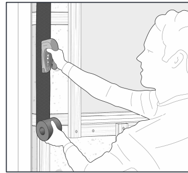
Cover all battens with EPDM strip
