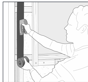
Cover all battens with EPDM strip
